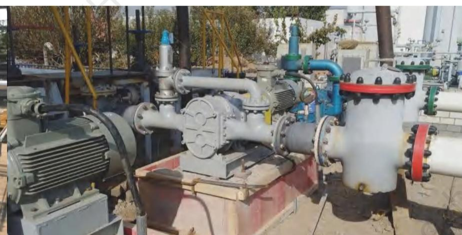
Lobe Pump (with Basket Filter and Safety Valve) Application to Chemical Industry
